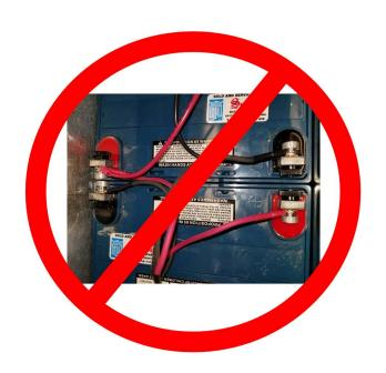
5. **Never** install batteries with the terminals facing each other.
